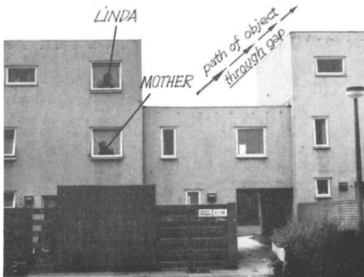
Photo 1: The closeness of the passage through the gap.
