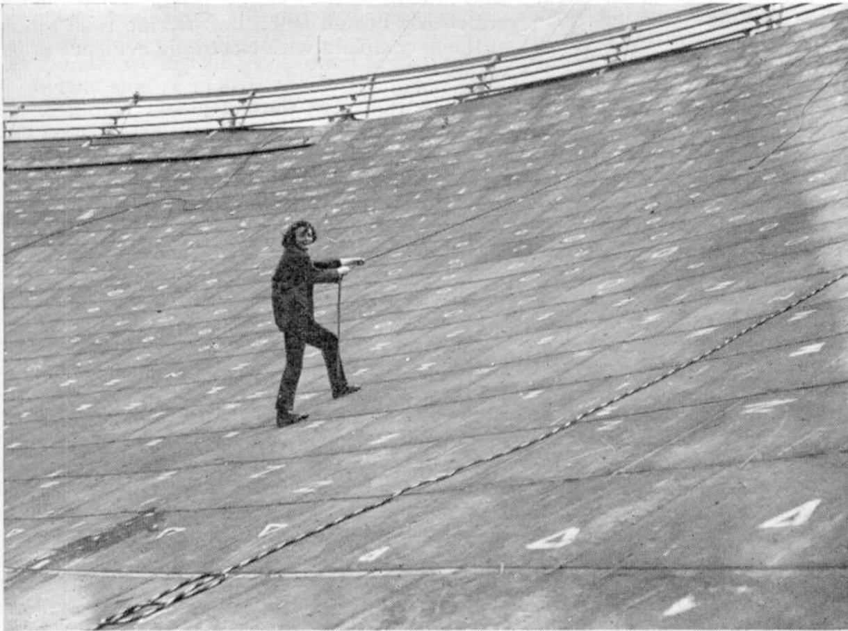
Some idea of the giant size of the telescope can be gained from this photograph of a girl climbing the wide open spaces of the curved reflector bowl. Built on a cradle of steel scaffolding, it has 7,000 steel plates, each separately welded.
